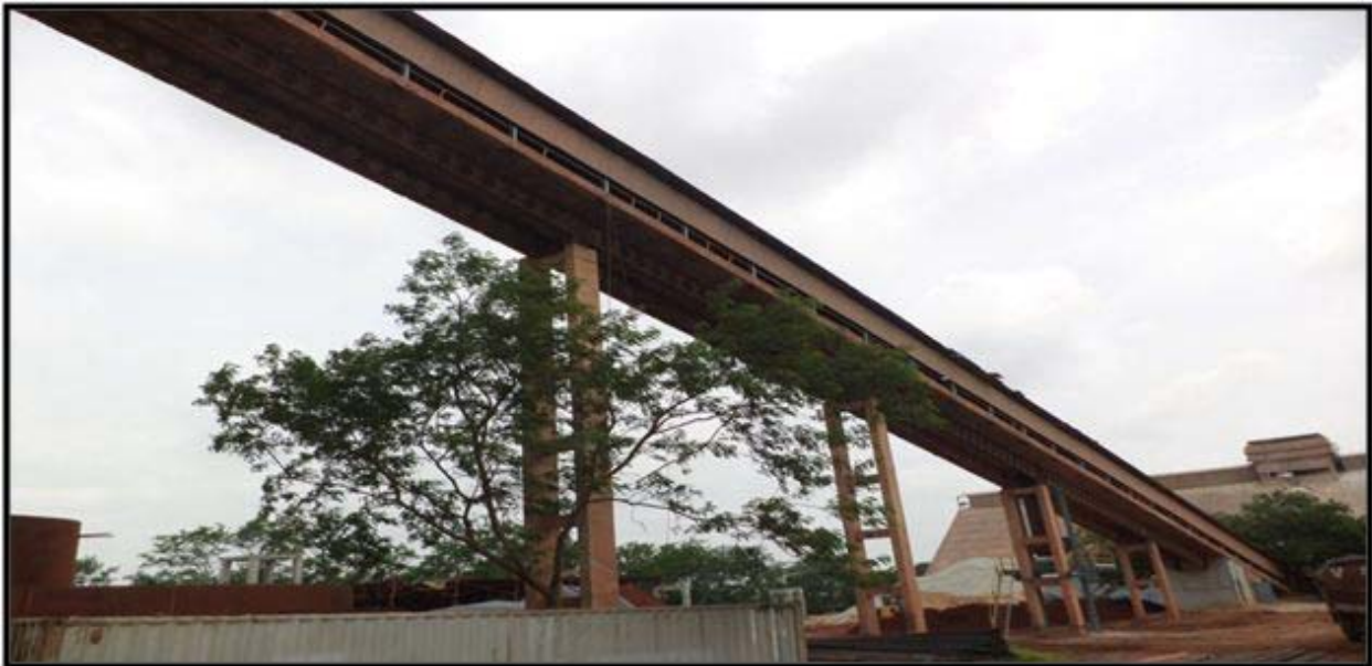
Covered belt conveyores
