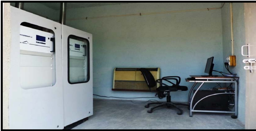
CAAQMS Station-3 installed at Mines area
