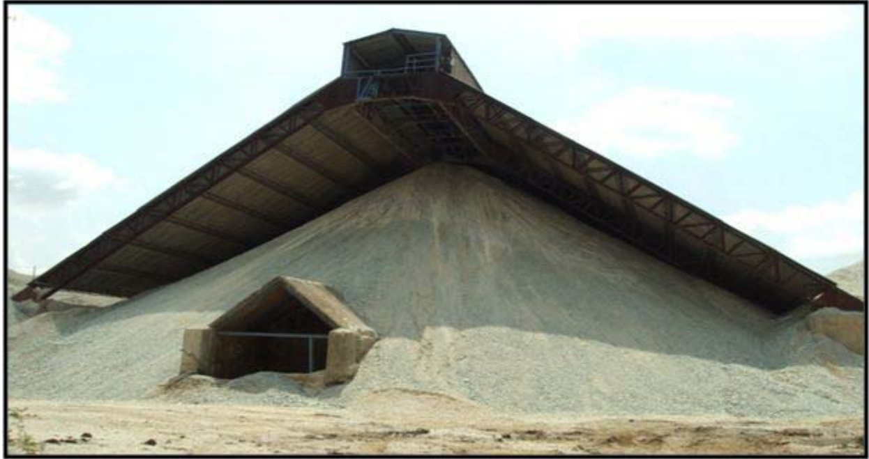
Crushed lime stone yard
