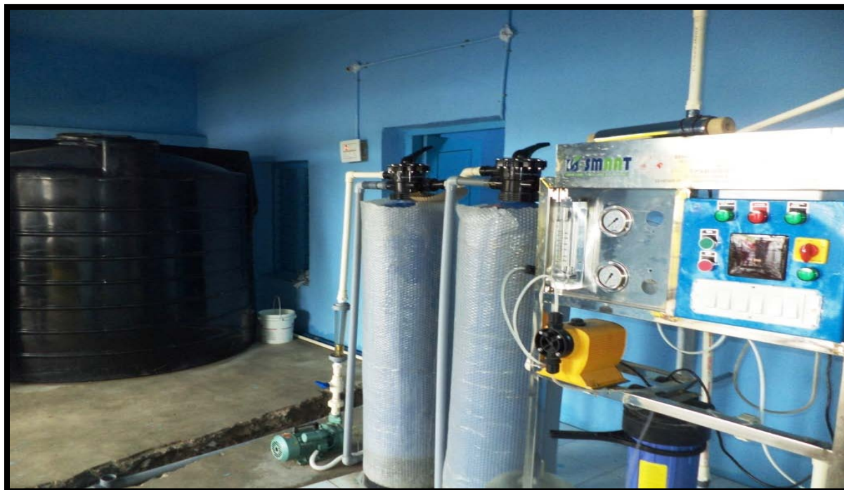
RO Water Plant Provided in Srinagar village
