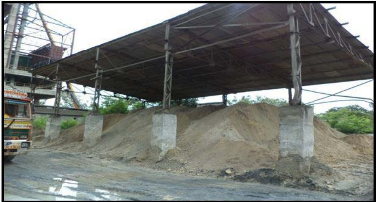
Coverd Gypsum yard
