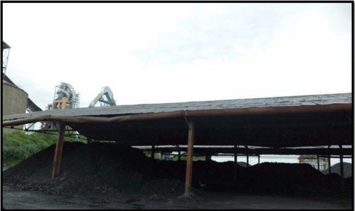
Covered Coal yard
