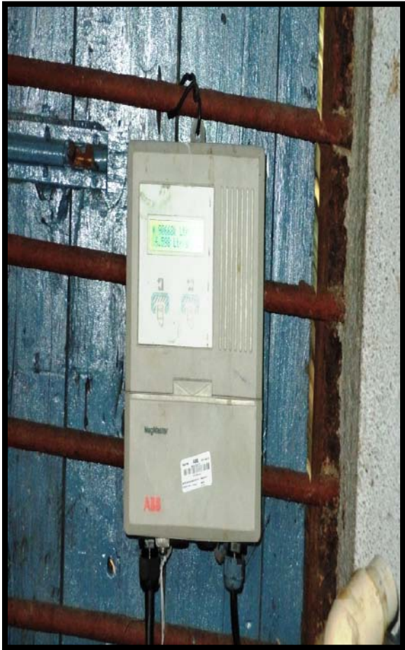
Colony Water meter,
