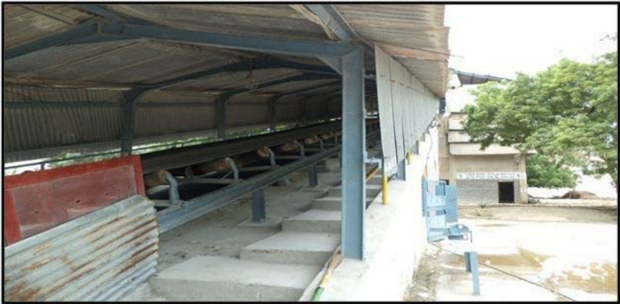
Covered belt conveyores
